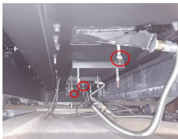
EX 2: AIR SHUTTER ADJUSTMENT UNDER YOUR FIREPLACE
